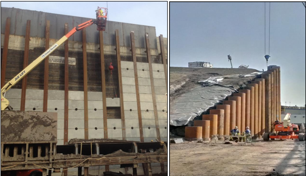
MSE Front Wall and Wing Wall
